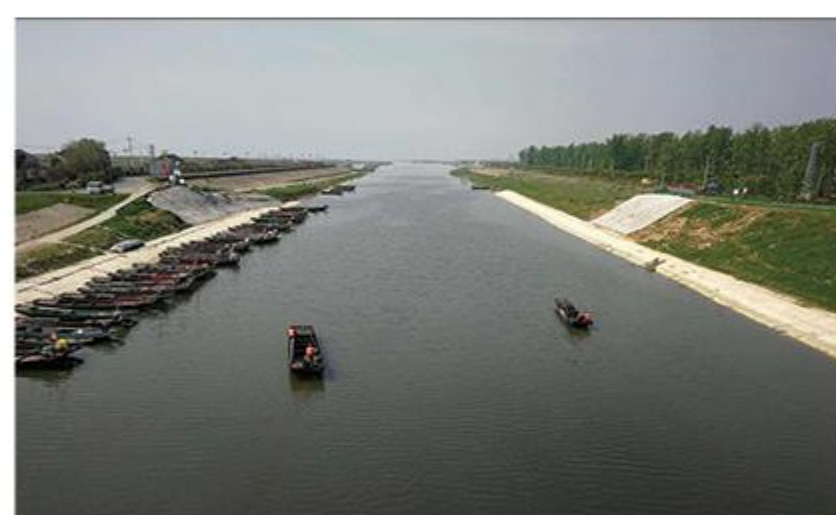
Channel obstruction detection
